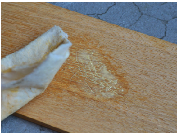
Re-oil with Rubio Monocoat hard wax oil
